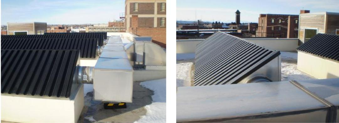
Figure C-3: Demand-based ventilation system with solar duct preheat, Orange Crush Building, Great Falls Montana
