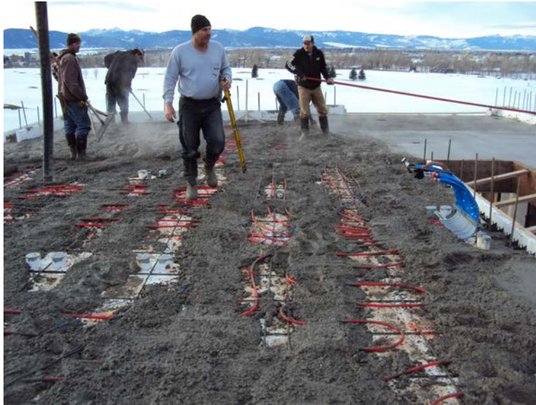
Figure 17. Over poured concrete slab with embedded 1/2" PEXa pipe
