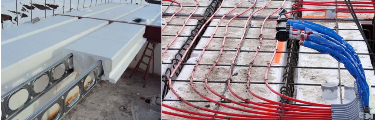
Figure 16. Different phases of the floor construction
