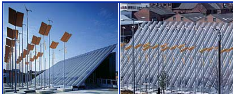
Hull Architecture Centre, Hull, England Níall McLaughlin Architects created a zero-energy temporary structure to raise design awareness in Hull. Wind turbines and photovoltaics mounted in a plaza supply the building’s energy and feed back into the city’s grid. Photography: © Nick Kane
