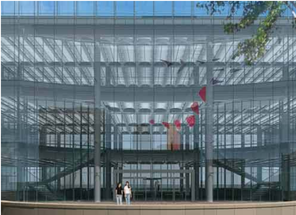
A library at Chicago’s Loyola University uses a double-skinned glass curtain wall.
